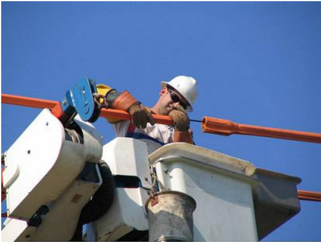
Tom Miller installing high voltage line hose at Letterkenny Army Depot
